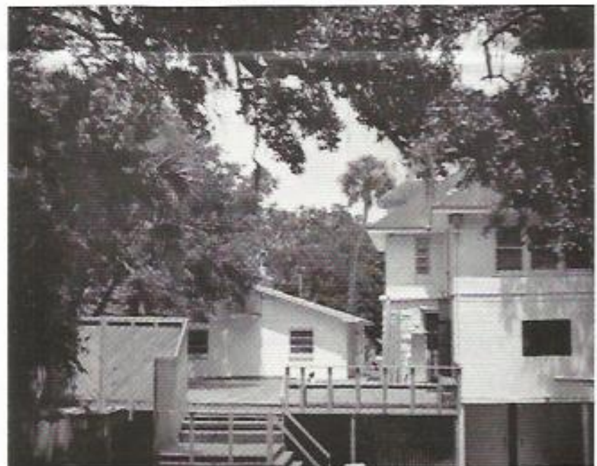
The Deck Nears Completion !!!
